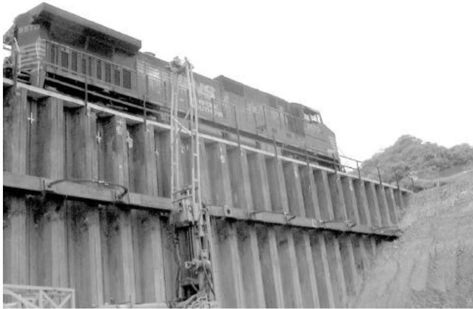
FIG 2. Shoring Wall Under Railway Loading
