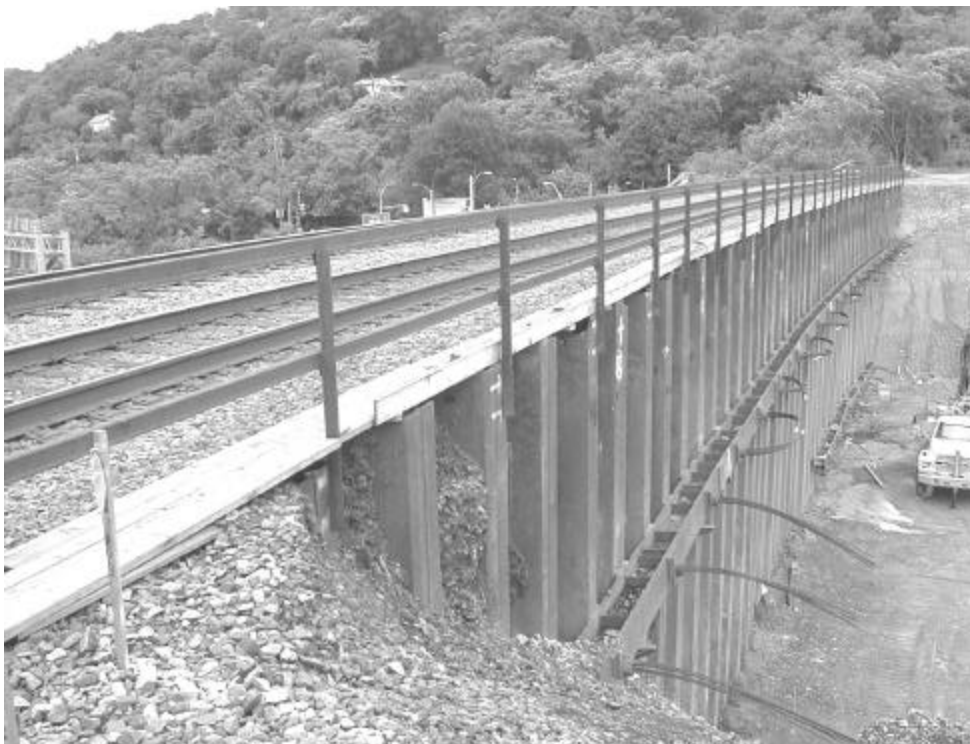
FIG 3. Shoring Wall After Installation of Level 2 Ties
