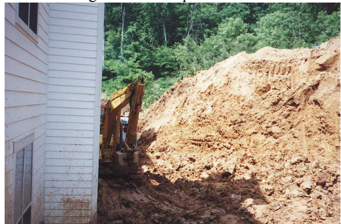
Figure 8. Emergency excavation of slide material
