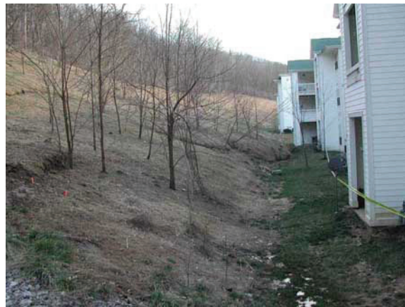
Figure 2. Early warning signs, small bulges in the slope.
