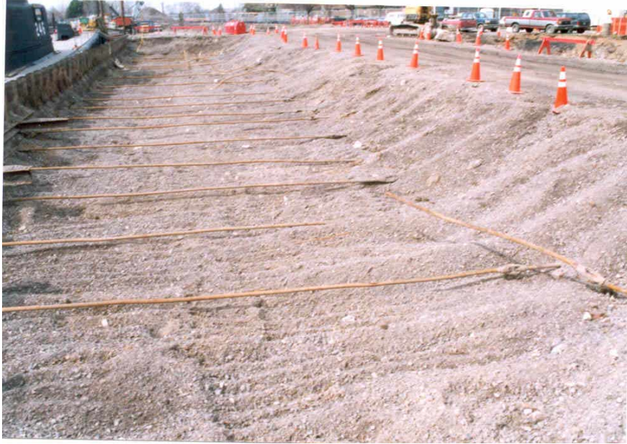
FIGURE 9 Thirty-three Year Old Bars, Backfilled in Free Draining Gravel Behind the Old Quay Wall, and Unearthed at the Buffalo Inner Harbor Project
