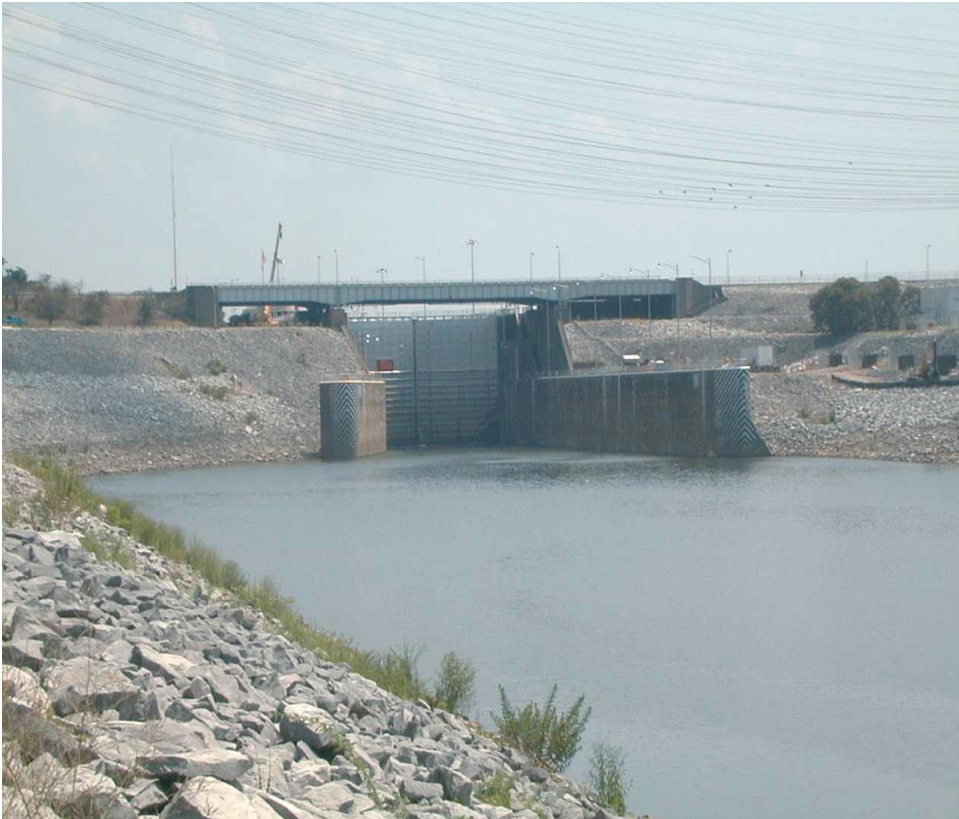
Downstream entrance to lock chamber at Kentucky Lock.
