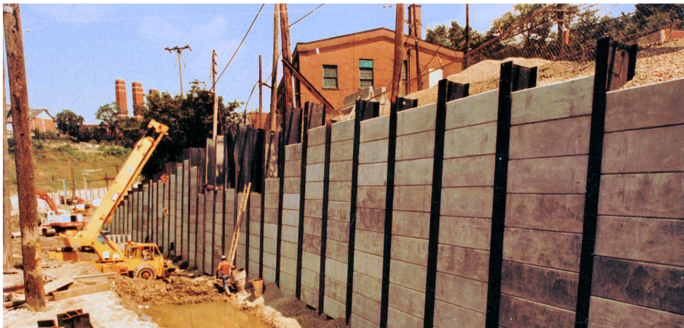
Soldier pile and concrete lagging retaining wall along LRT above-ground alignment.
