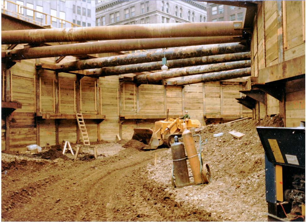
*Braced excavation for construction of the Gateway Center subway station in Pittsburgh.*
