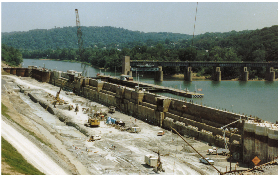
Excavation for new lock and instrumented existing lock monolith wall.
