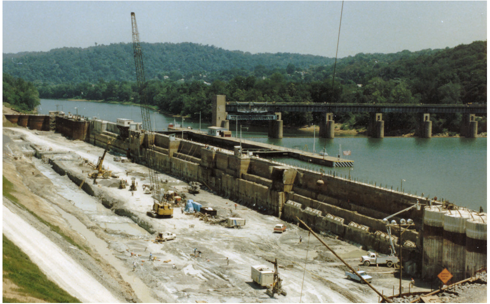
Excavation for new lock and instrumented existing lock monolith wall.
