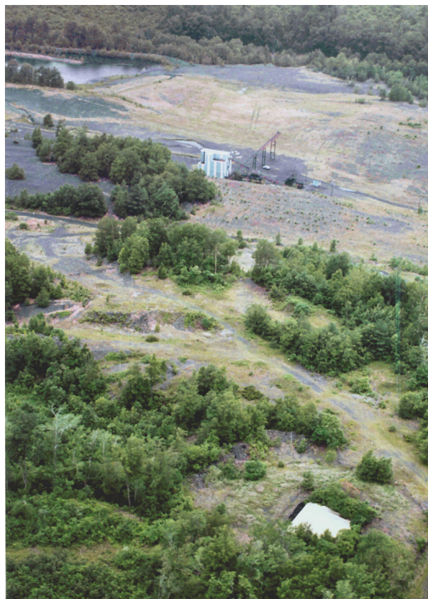
Aerial view of the Blackwood Mine Site at the time of the study. The building is an abandoned coal breaker. The square concrete pad in the foreground covers a deep ventilation shaft to the mine, but the sides of the pad partially collapsed, requiring further remediation.
