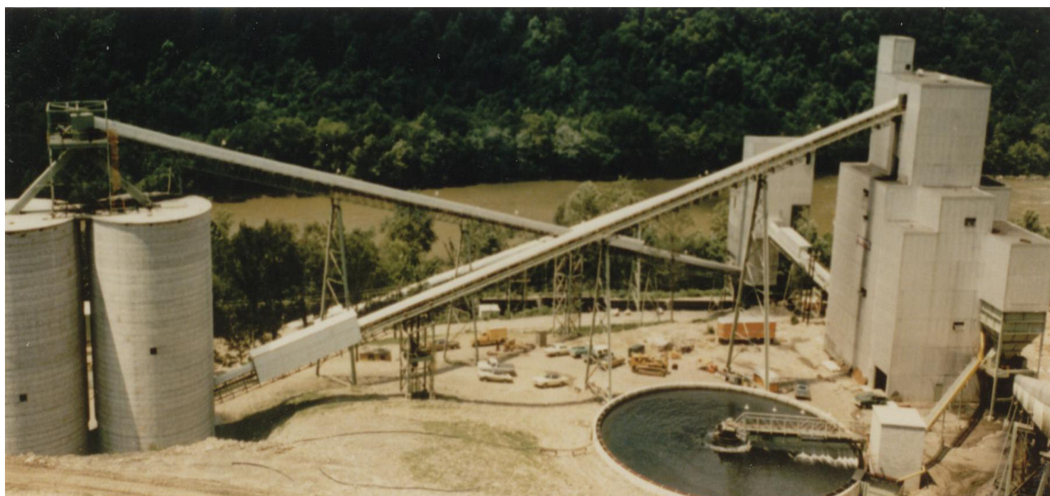
Major site structures for coal preparation complex located in the New River Gorge.
