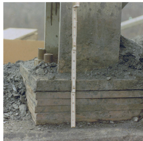
Shims placed beneath column supports for a 100-ton storage/truck loading bin.
