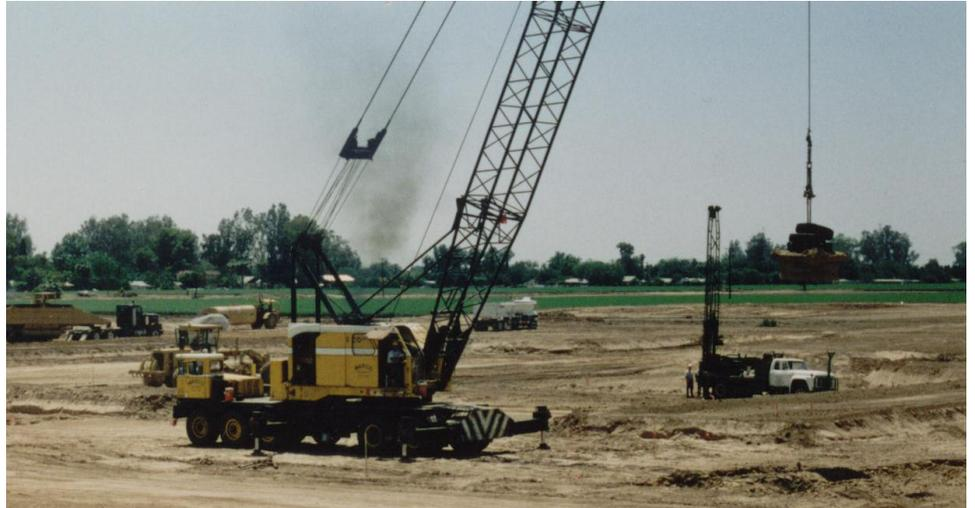
Crane lifting 13-ton weight prior to drop. SPT tests being performed on compacted area.
