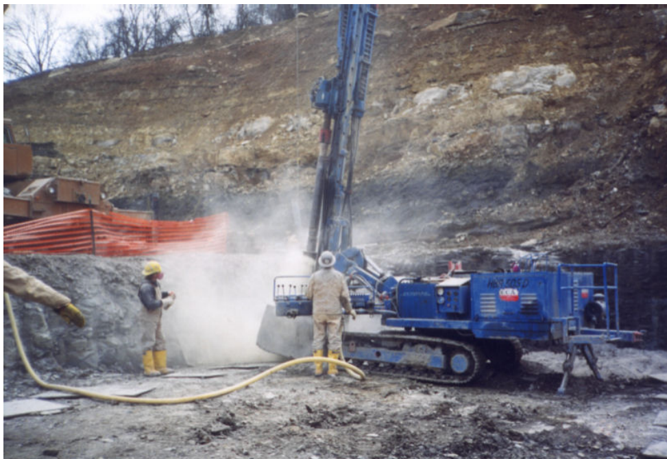
Installation of 12-inch-diameter pipe piles recommended in D'Appolonia's VE design.
