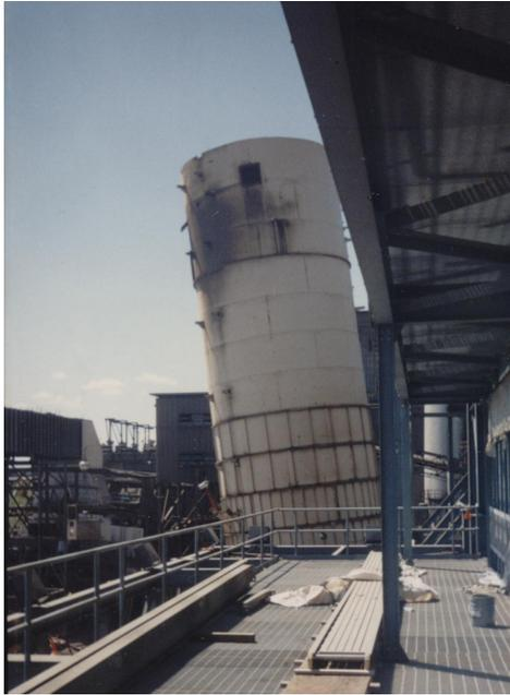
Storage tank exhibiting tilt resulting from foundation failure caused by collapse of subgrade cooling pipes.
