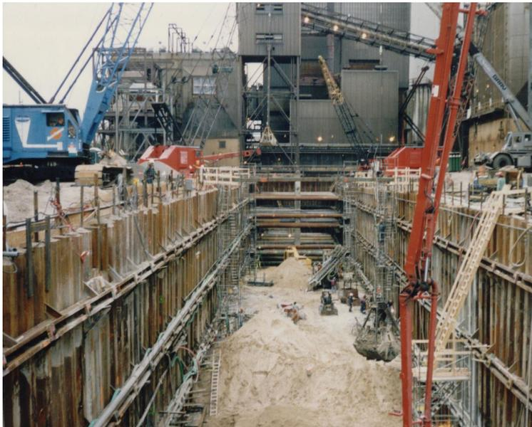
Sheet pile wall used for ground support during replacement of failed 14-foot-diameter cooling pipes located 60 feet below grade.
