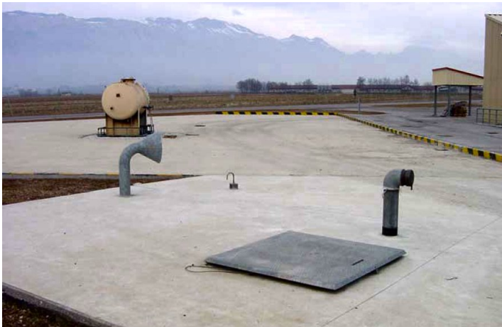
Stormwater control structures at the Aviano Air Base.
