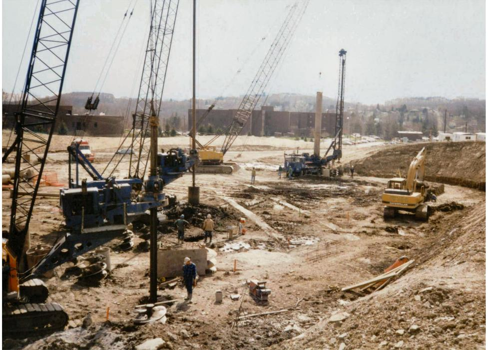
*Construction of cast-in-place, reinforced concrete drilled shafts through mine spoil and foundation preparation for the MSE retaining wall. Temporary casings were installed through the mine spoil to prevent caving and to facilitate construction and monitoring.*
