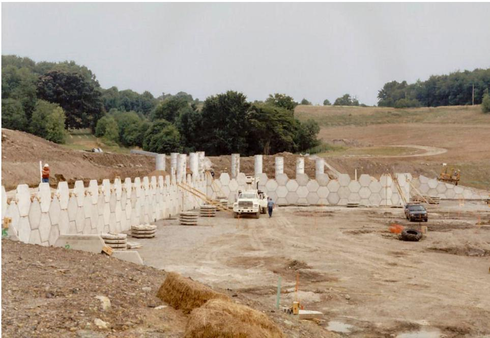
*MSE retaining wall construction immediately adjacent to the building footprint. Casings behind the retaining wall facing were used to isolate drilled shafts for foundation support from the reinforced soil fill and to reduce downdrag forces from mine spoil consolidation.*
