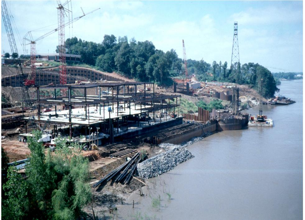
*Ameristar Casino during construction of the enclosing cofferdam. The two-tiered retaining wall system can be seen in the background.*
