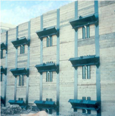
*Anchored soldier pile and lagging retaining wall system.*
