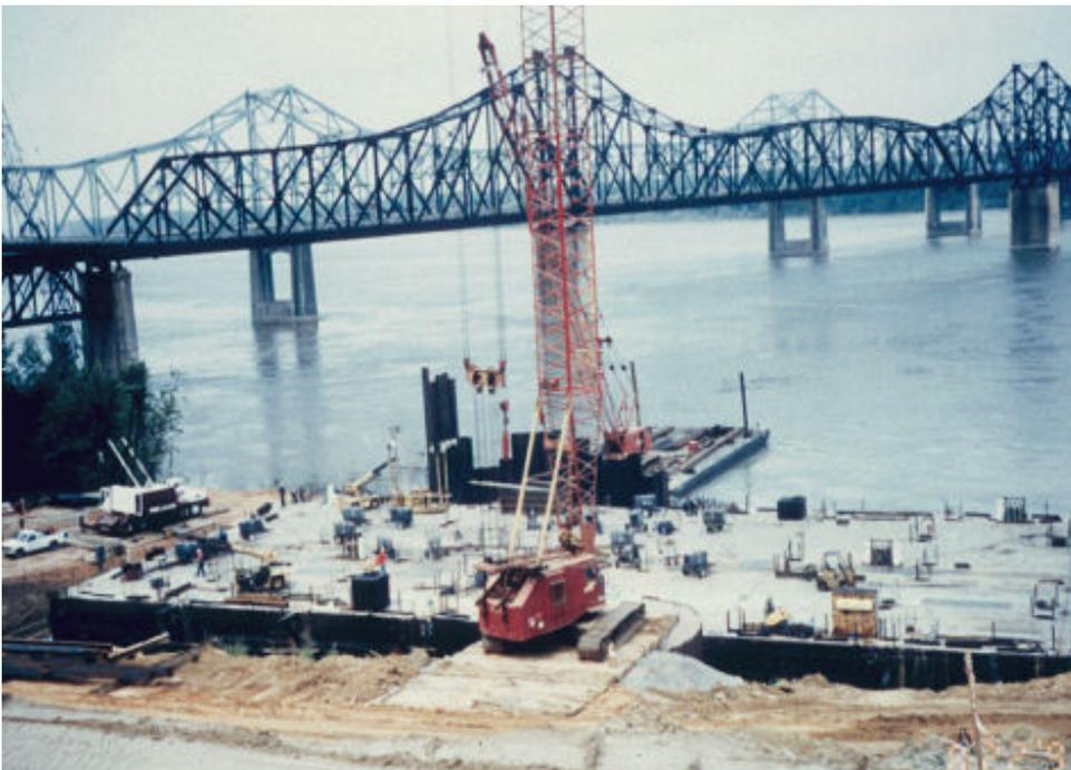
*Construction was conducted from both land- and barge-mounted equipment.*
