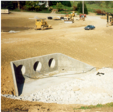
Dam and spillway nearing completion.
