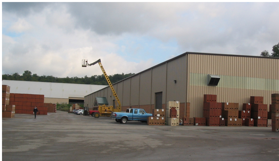
New structures and brick storage at the Redland Brick manufacturing plant.
