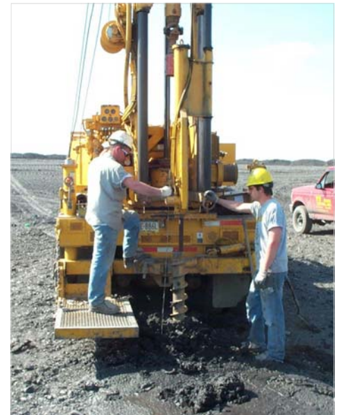
Drilling activity at one of the two platform locations.
