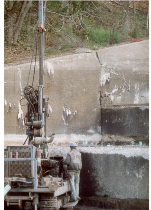
*Anchor installation at spillway step.*
