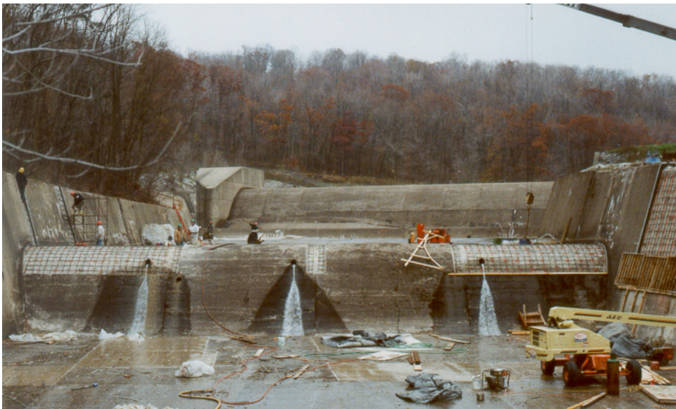
Rehabilitation work in progress on the Quemahoning Dam emergency spillway.
