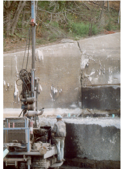
Anchor installation at spillway step.
