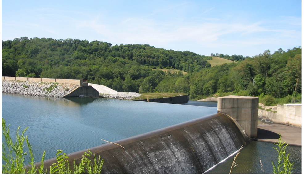
Raised crest and new armored spillway channel embankment at Quemahoning Dam.
