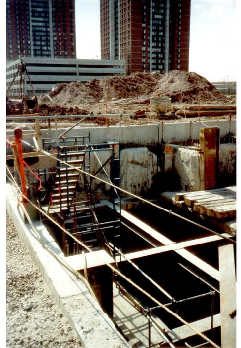
*Top of shaft showing perimeter diaphragm wall and internal bracing.*
