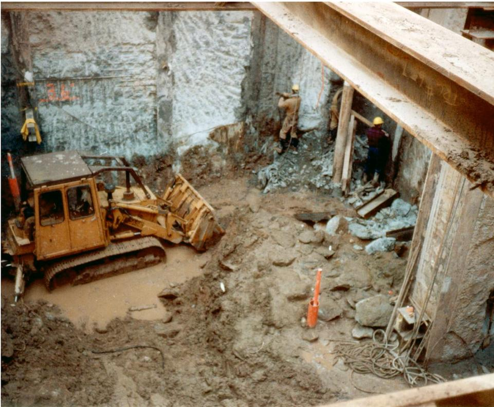
*Excavation of rock inside 60- by 63- by 80-foot-deep shaft.*
