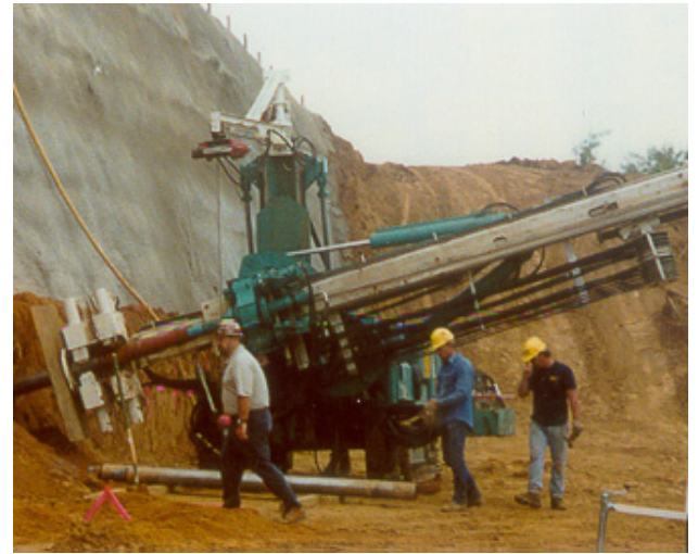
Soil nail installation at Natchez Bluff site.
