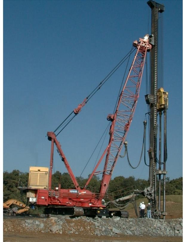
*Deep soil mixing with triple five-foot-diameter augers.*
