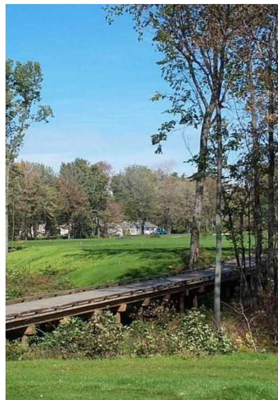
View of Millcreek Golf Course following site remediation and redevelopment.
