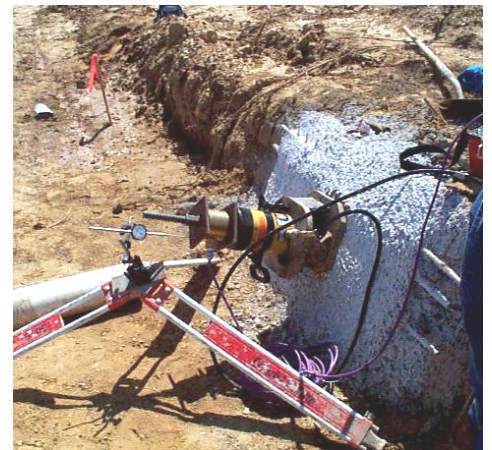
Pre-production soil nail load test.
