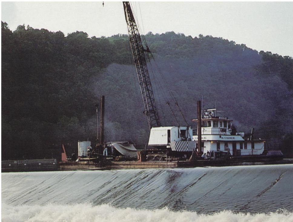
*Drilling conducted from barge in the Allegheny River to obtain core samples from a concrete dam and samples of subsurface foundation soils.*
