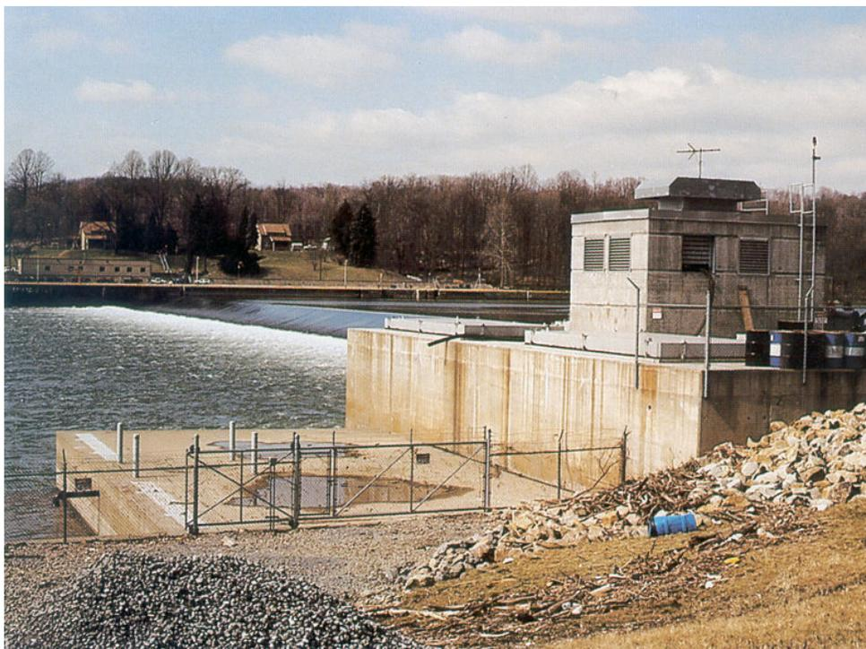
*Completed 12-MW, low-head hydroelectric generation plant on the Allegheny River.*
