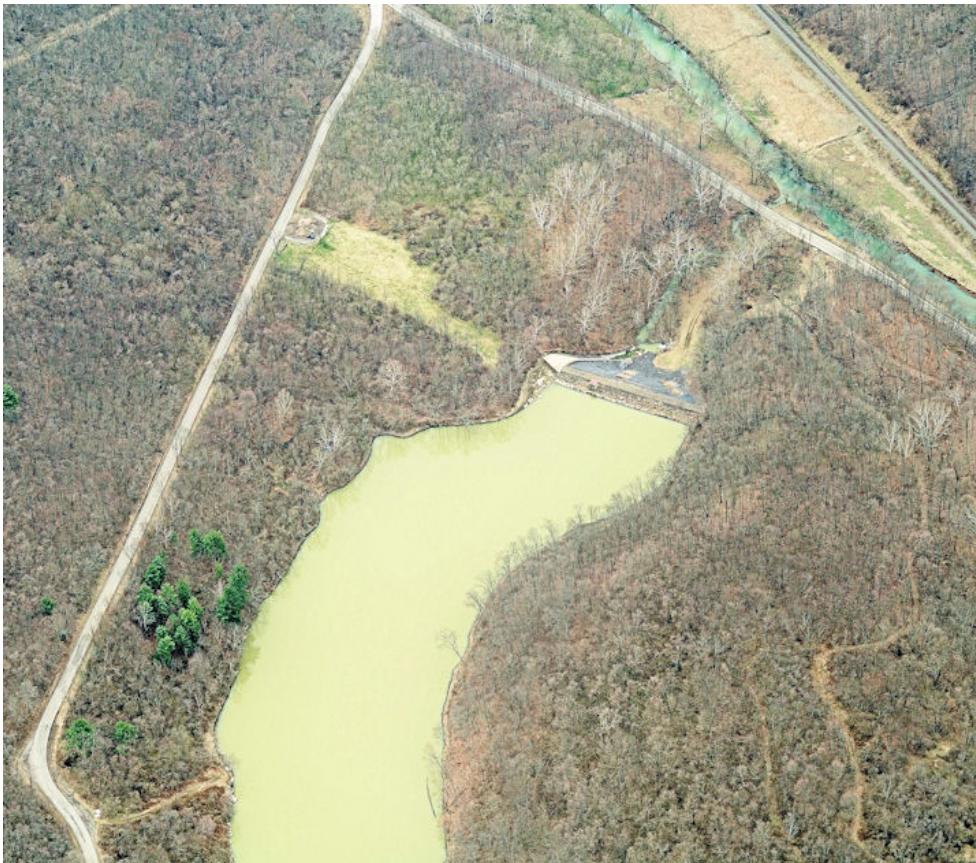
Aerial view of Wisecarver Dam and associated spillway and impoundment.
