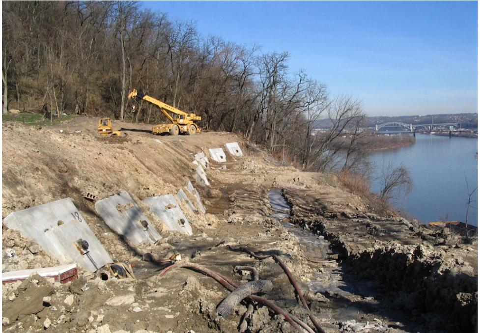
*Slope at Corfu Street during installation of ground anchors and surface reaction pads.*
