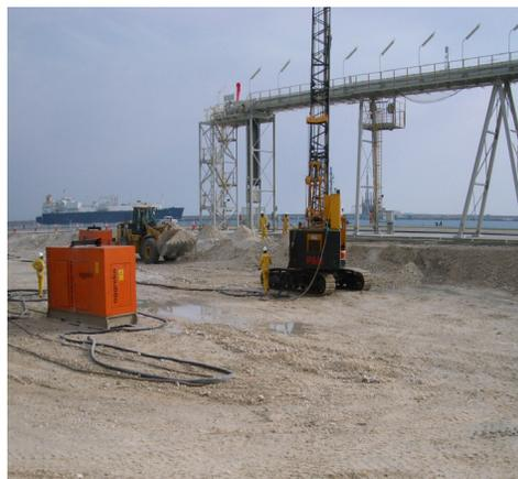
*Vibro-compaction at the CSP site. Note the power generator to the left of the rig.*
