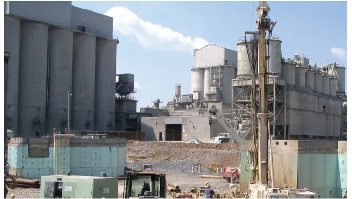
Micropile installation for Finish Mill foundation.
