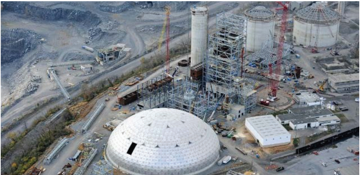
Aerial view of $400 million cement plant expansion.
