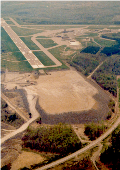
Runway extension at Broome County Airport near Binghamton, New York.
