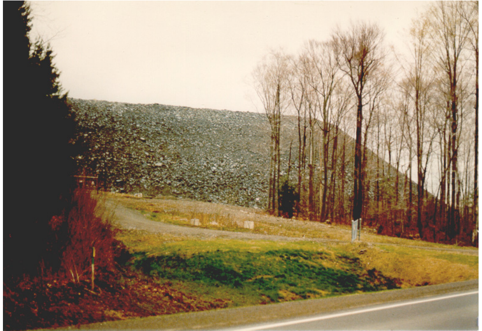
Runway extension fill viewed from adjacent highway.
