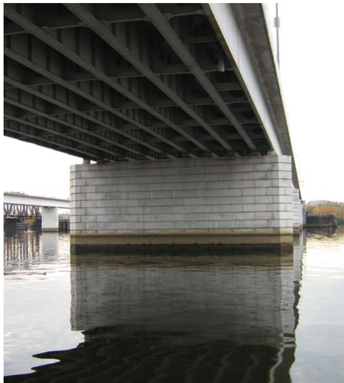
Pier at the 14th Street Bridge in Washington, DC.
