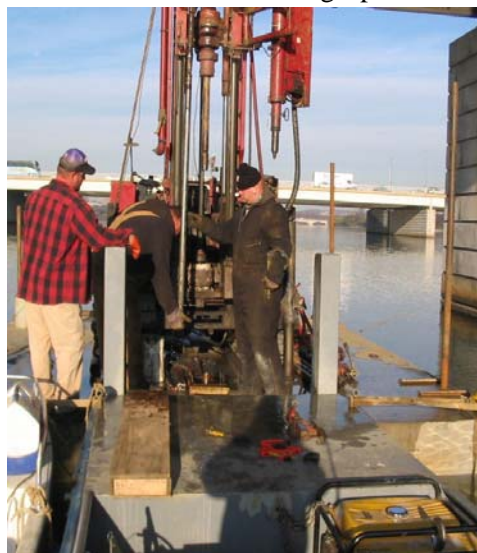
Drilling activities adjacent to bridge pier.
