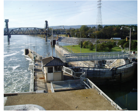
Chickamauga Lock on the Tennessee River. issues associated with difficult geotechnical conditions at the site.
