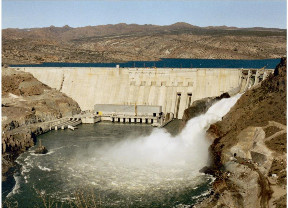
The Piedra del Aguila Hydroelectric Project including dam, spillway and generating plant.
