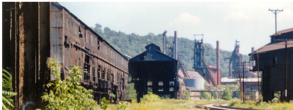
These structures were demolished as part of environmental remediation, allowing for conversion of this riverfront property into a light-industrial park.
