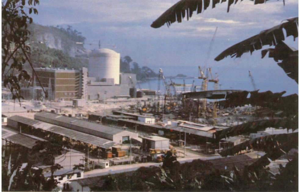
The Angra Nuclear Power Plant during construction.
