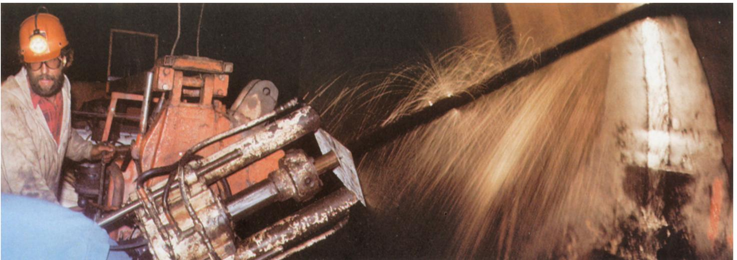
*Drilling of 30-foot-deep, three-inch-diameter boreholes through tunnel liner into rock.*
